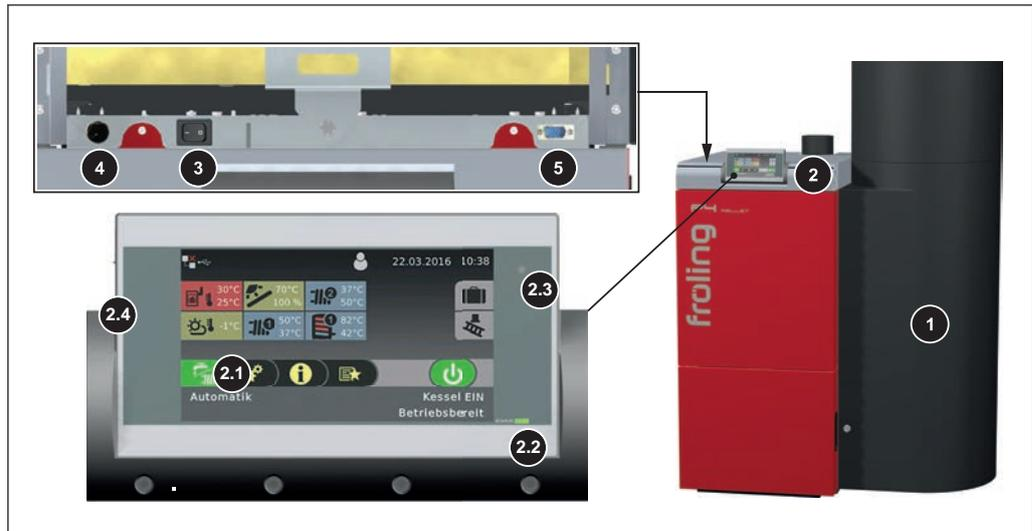
1 P4 Pellet with integrated pellet cyclone container
